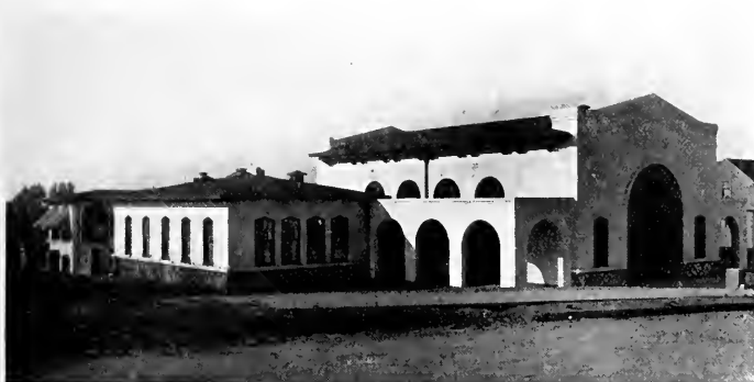
FRONT VIEW, CLEVELAND SCHOOL, OAKLAND John J. Donovan and Shafer & Wilde, Associate Architects
